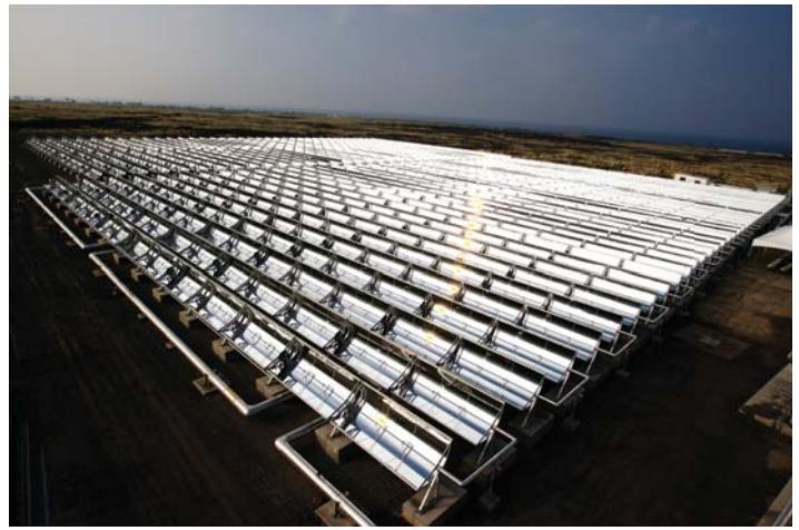
An image of MicroCSP collectors on the Big Island of Hawai'i. Source: Wikipedia
